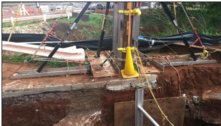
Using 2 Ver-T-Pols with only 2 legs on each unit
