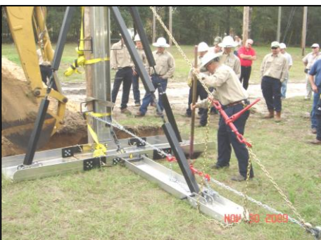
Removing sand from underneath base
