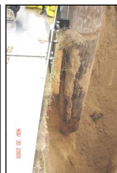
Pole butt free floating
