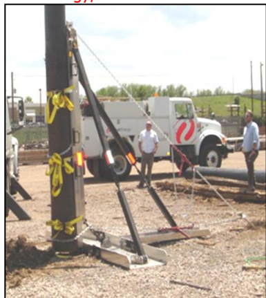
Pole attached to free standing Ver-T-POL
